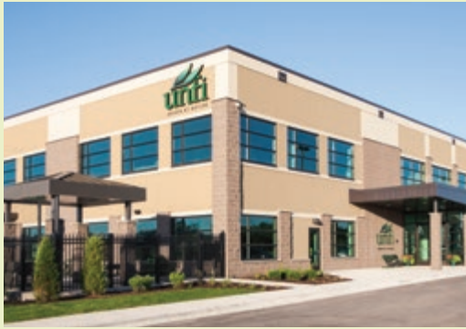
RACINE, WISCONSIN LEED® Gold Certification Expected
