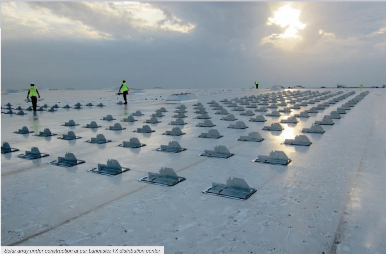
Solar array under construction at our Lancaster, TX distribution center
